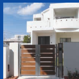
門扉設置・取替
