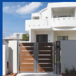
門扉設置・取替
