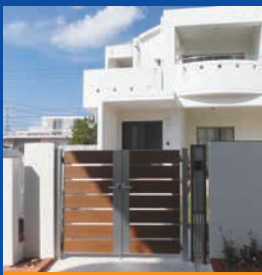
門扉設置・取替
