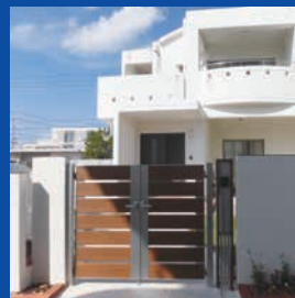
門扉設置・取替
