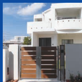
門扉設置・取替
